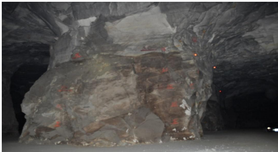
Figure 1.6A 12.192 square meter pillar size and 9.144 m high; room width of 10.36 m; pillar life is over 60 years; overburden depth is 57 m.
